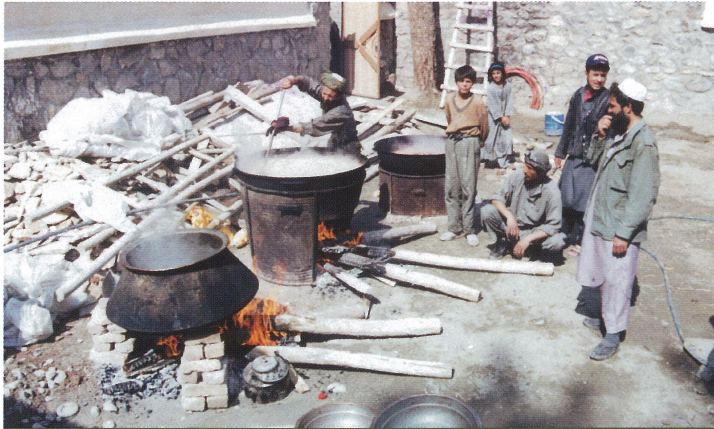
Members of the 90-person crew wait for lunch to finish stewing in the vats. The crew often used this outdoor kitchen to cook large meals on the construction site.
