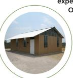
expensive to construct. The One-Day School is an effective solution. A kit comes with a steel roof and walls, windows, doors, and desks.
